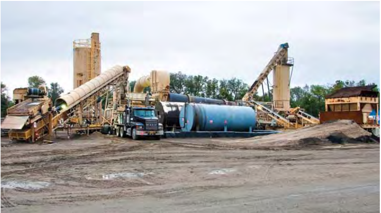
Yates, which operates three asphalt plants and three paving crews out of Jackson, MS, was able to increase production by about 300 tons a day as a result of the Trimble PCS400 Paving Control System.
